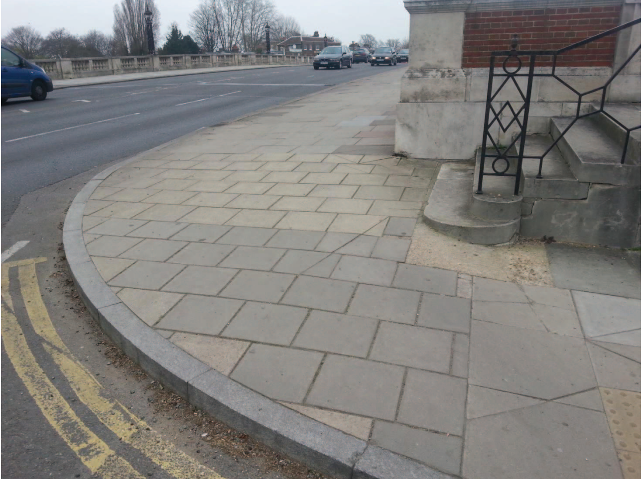
Photo B – from Cigarette Island looking north over Hampton Court Bridge from location where most pedestrians cross the carriageway in-line, with improved visibility to the north.
